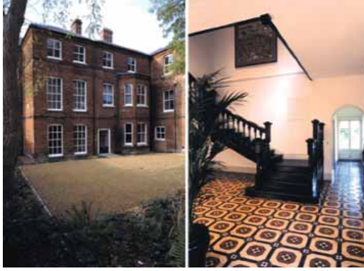
The Sainsbury Institute headquarters in Norwich
